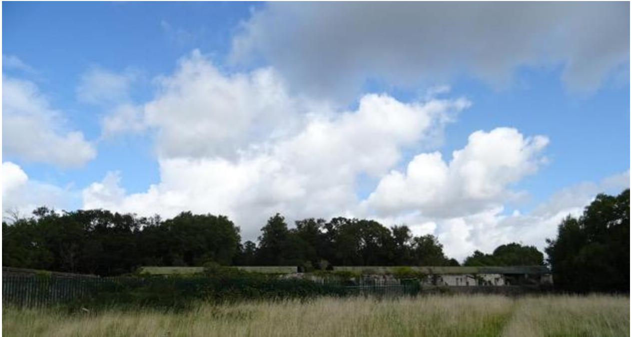
Fig.10: Non-historic fencing and concrete wall boundary wall at the south of the Coach House, proposed for demolition.
