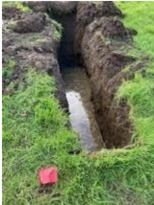
Plate 5 TP4 looking south.
