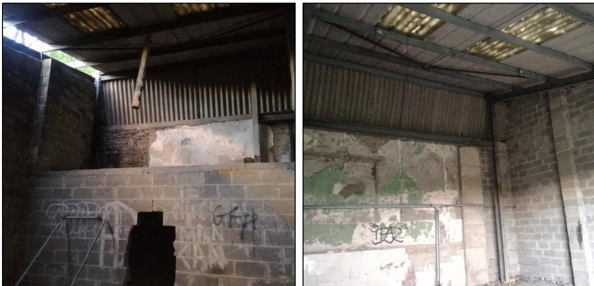
FIGURE 9. MODERN SHED BUILDING.
