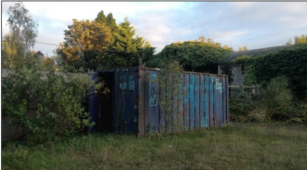
FIGURE 10. SHIPPING CONTAINER (STRUCTURE 'D').
