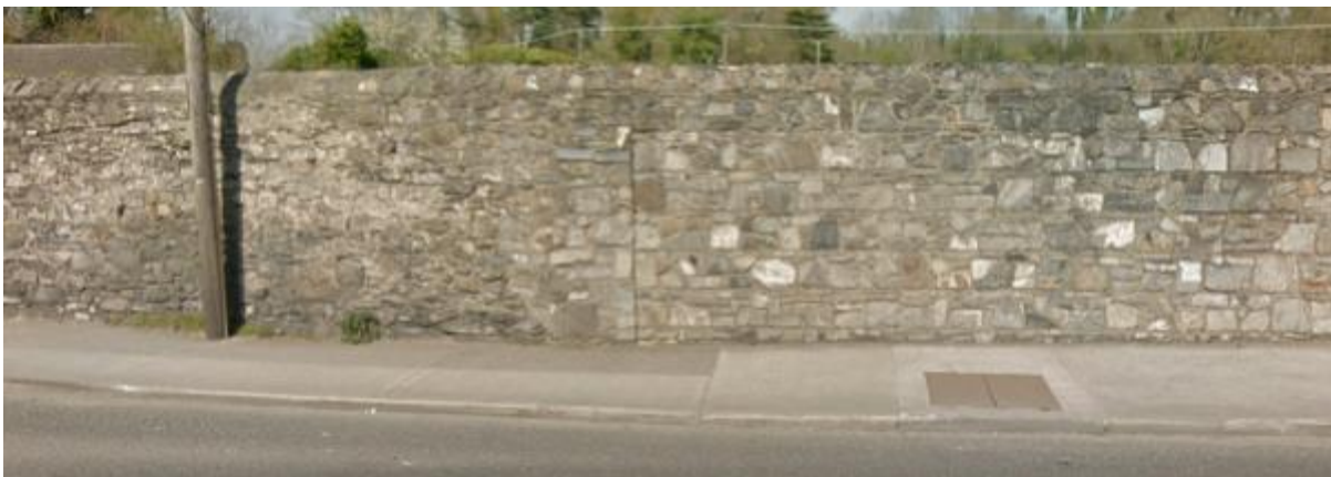
Figure 13 Elevation to Lucan Rd. Showing clear distinction in building methods.
