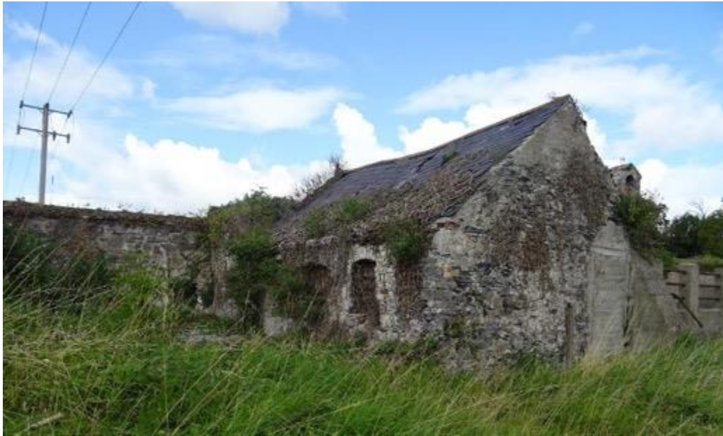
Fig.5: Historic Farm building proposed for demolition.
