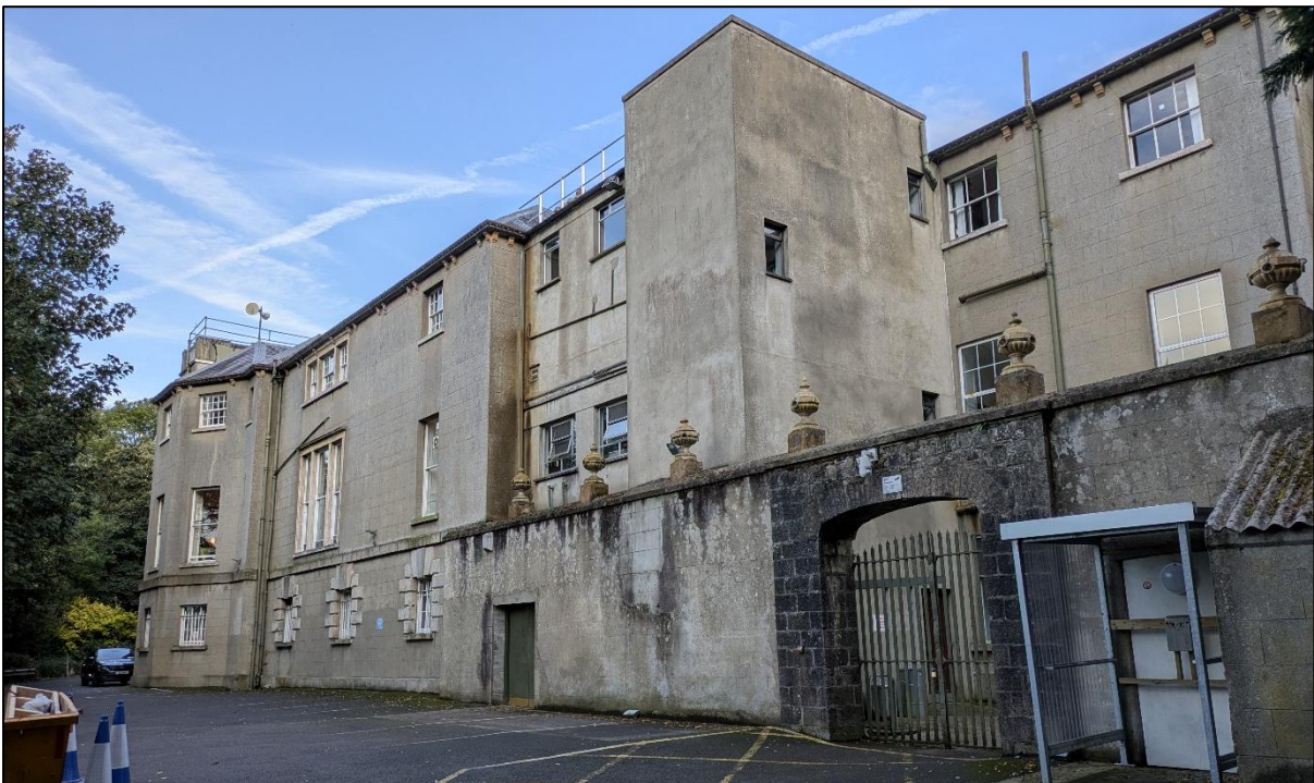
FIGURE 17. ST. PATRICKS HOSPITAL BUILDING REAR (STRUCTURE 'J').
