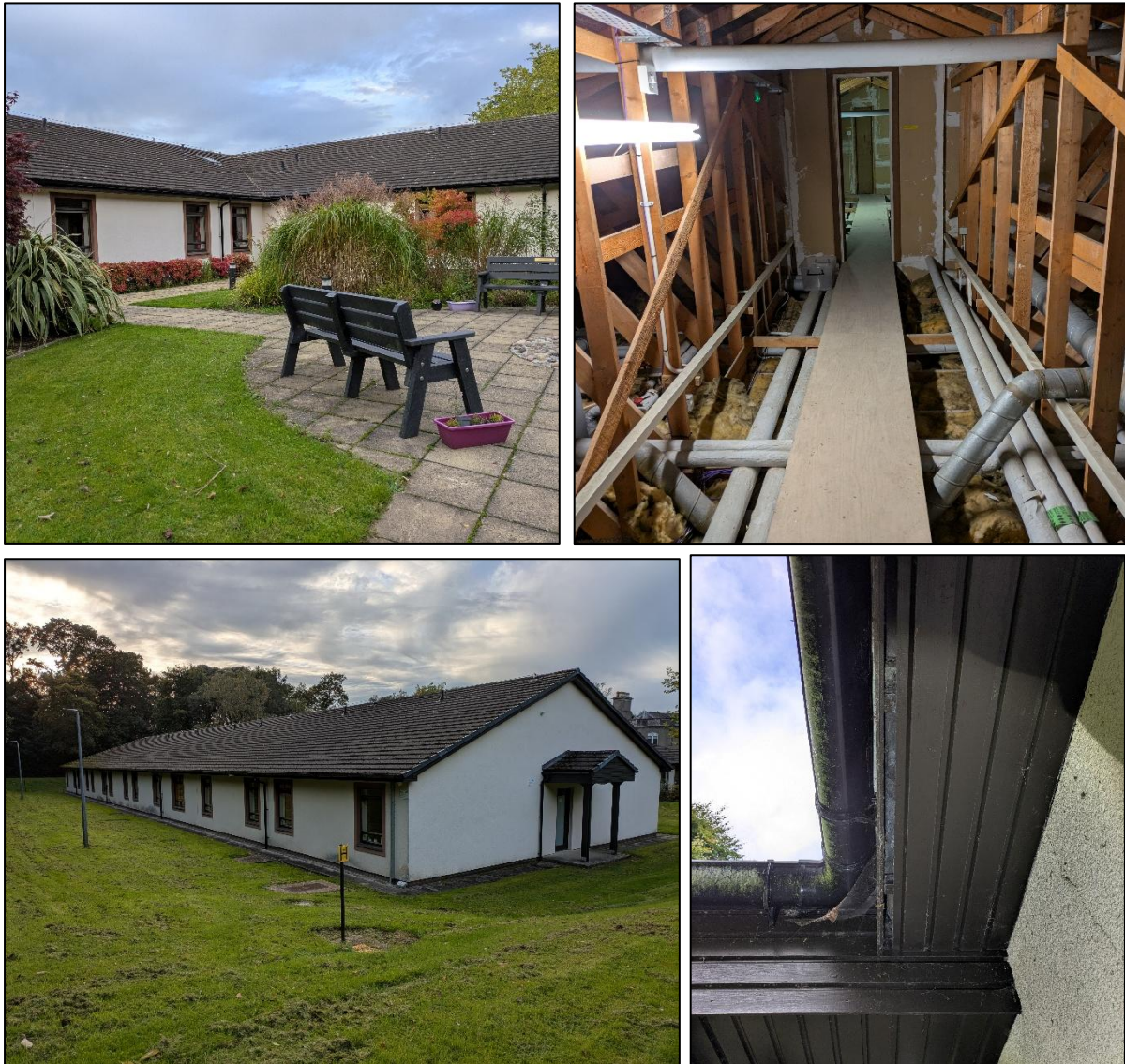
FIGURE 15. WARD (STRUCTURE 'I').
