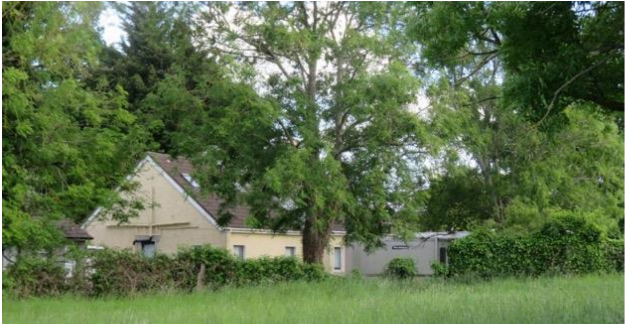
Fig.7: Non-historic bungalows buildings at the southeast of the site, proposed for demolition.
