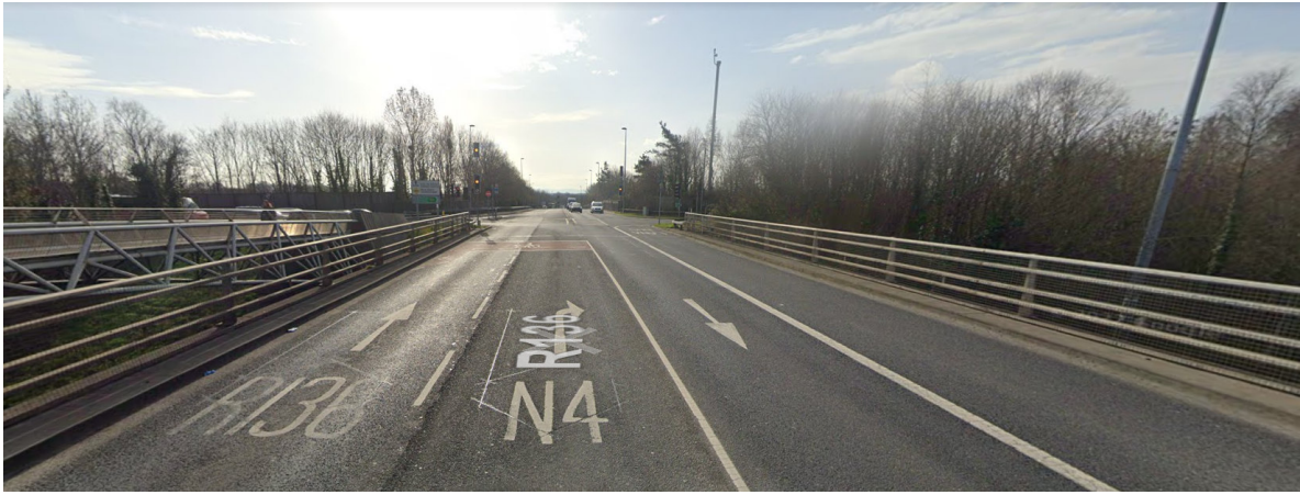
FIGURE 2.6 – JUNCTION 6 (R136/ N4 SLIP ROAD – WESTBOUND) (SOURCE: GOOGLE MAPS)
