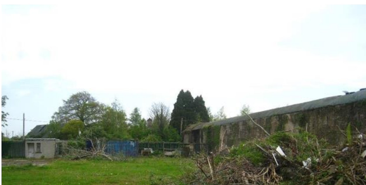
Fig.13: Non-historic ancillary building at the north of the Coach House, proposed for demolition.
